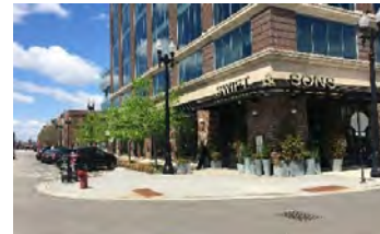
Curb Extensions / ADA Upgrades
