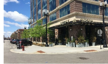
Curb Extensions / ADA Upgrades
